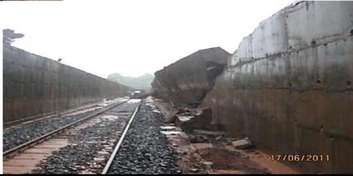
Slope Failure
