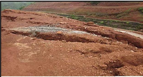
Raincuts due to erosion
